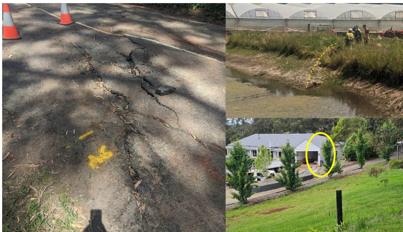
Figure 9: Recent infrastructure damage, Monbulk-Seville Road, Seville. Left: Damage to road. Top right: Landslide scarp through dam wall. Bottom right: Damage to property.
